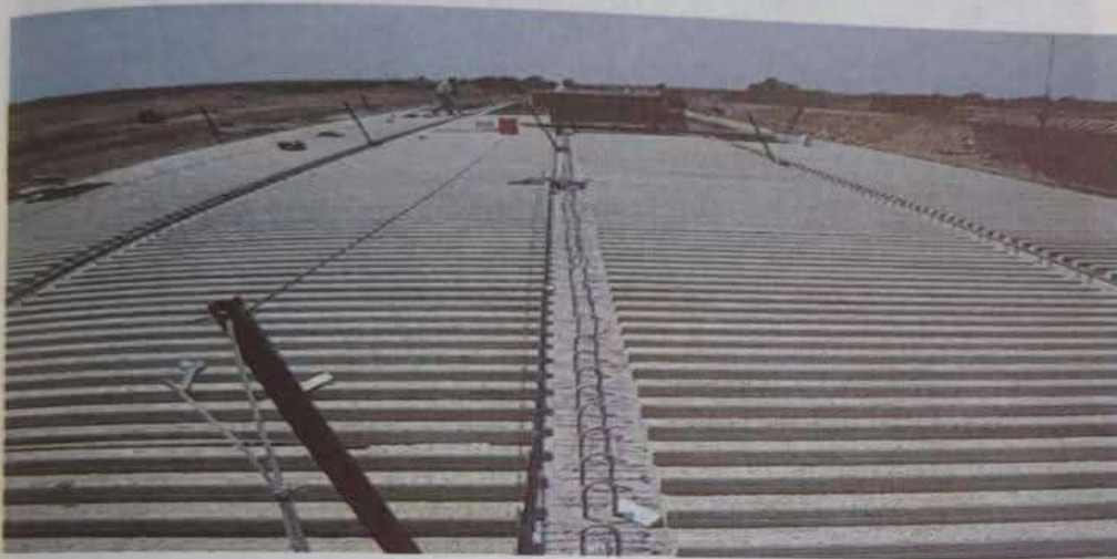
FIGURE 10.7 FRP deck panels over concrete girders [©Berg et al. 2006, reproduced with permission].
