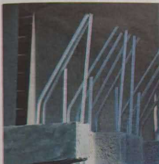
(a) Galvanized rebar in side barrier of a bridge
