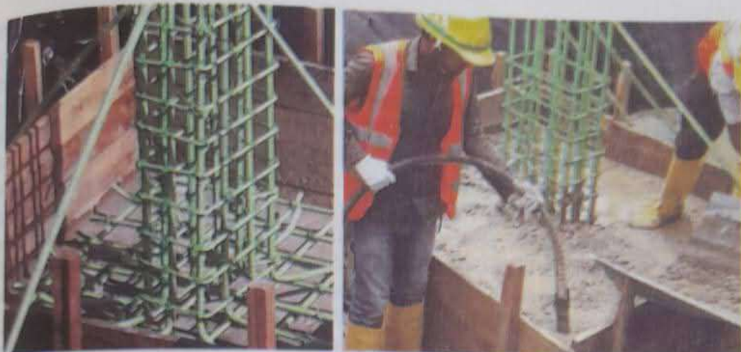
FIGURE 9.5 Application of ECR in a spread footing (Photo courtesy – BSRM).
