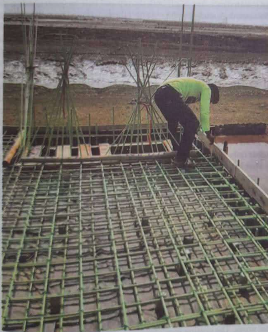
FIGURE 9.6 Application of ECR in floor slab (Photo courtesy – BSRM).
