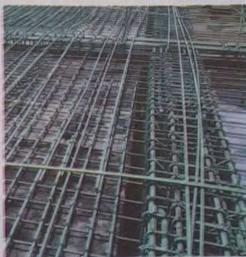
(b) Epoxy coated rebar on jetty deck (Photo courtesy - BSRM)
